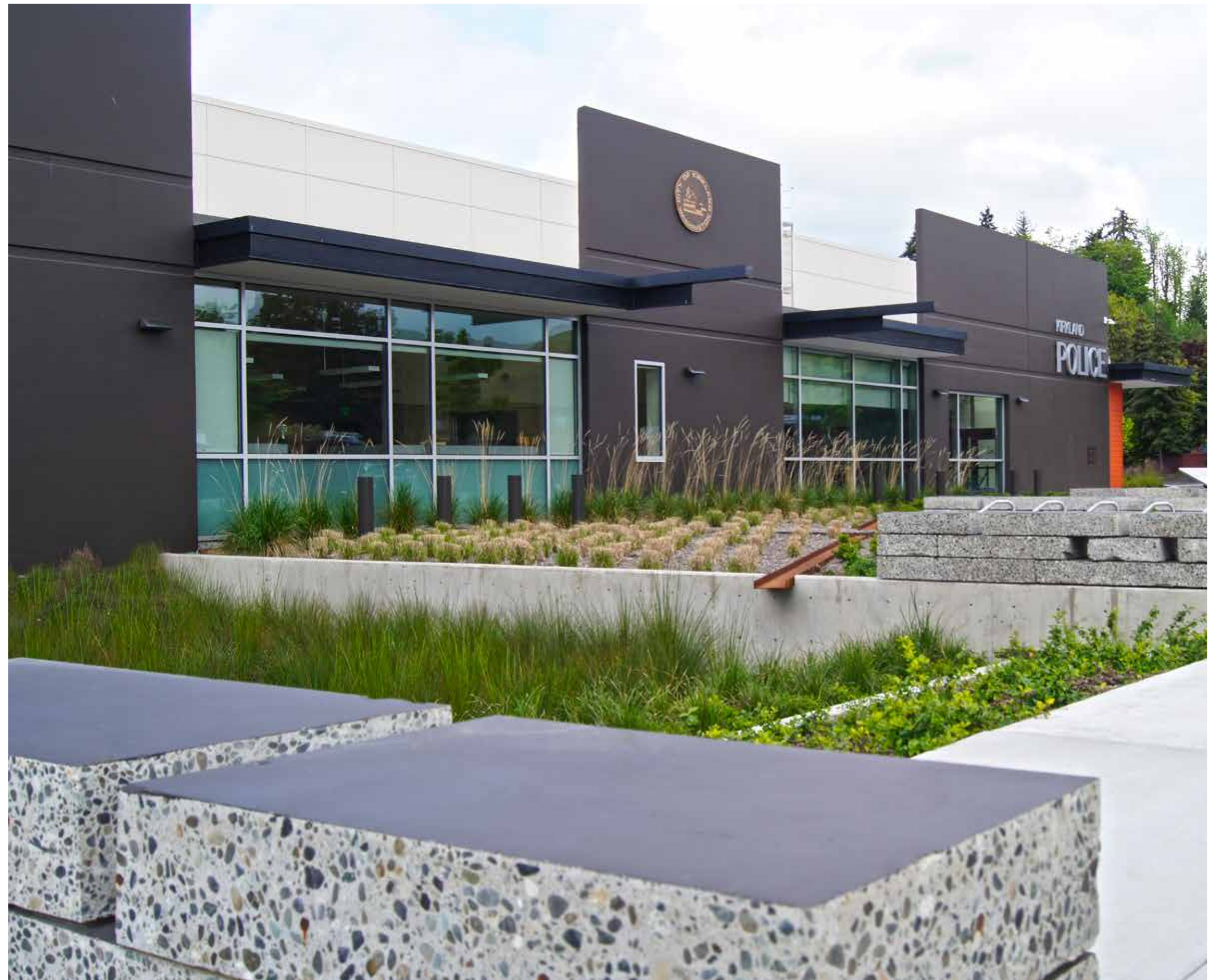
Repurpose Panels: Several sections of existing precast tilt-up walls were saw-cut into manageable sections then assembled into site walls. The walls provide seating opportunities and spatial definition adjacent to hardscape, but are also part of a subtle security measure.
