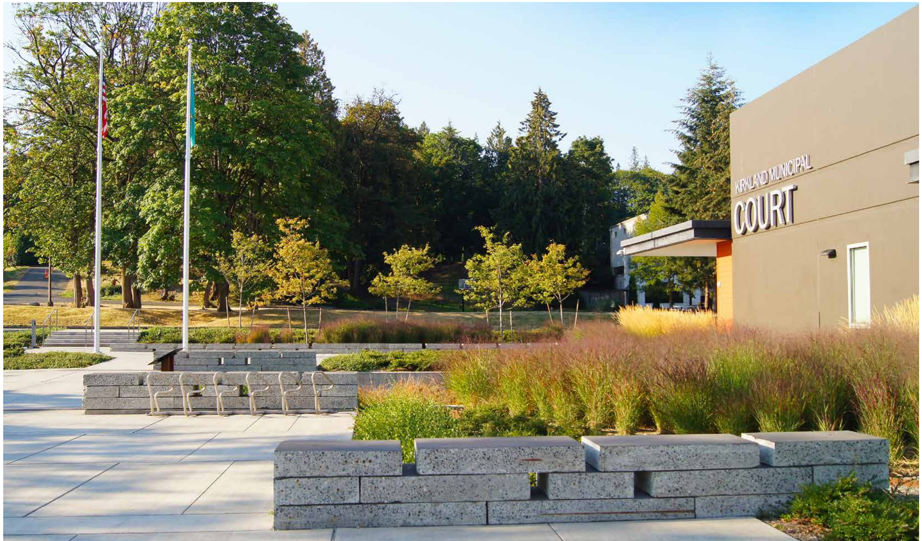
Site Walls: Aggregate and rebar were left visible to indicate second use of the reclaimed material, but top surfaces were painted and rubber shims provide shadow between layers to elevate the design of a humble, cost-effective material.
