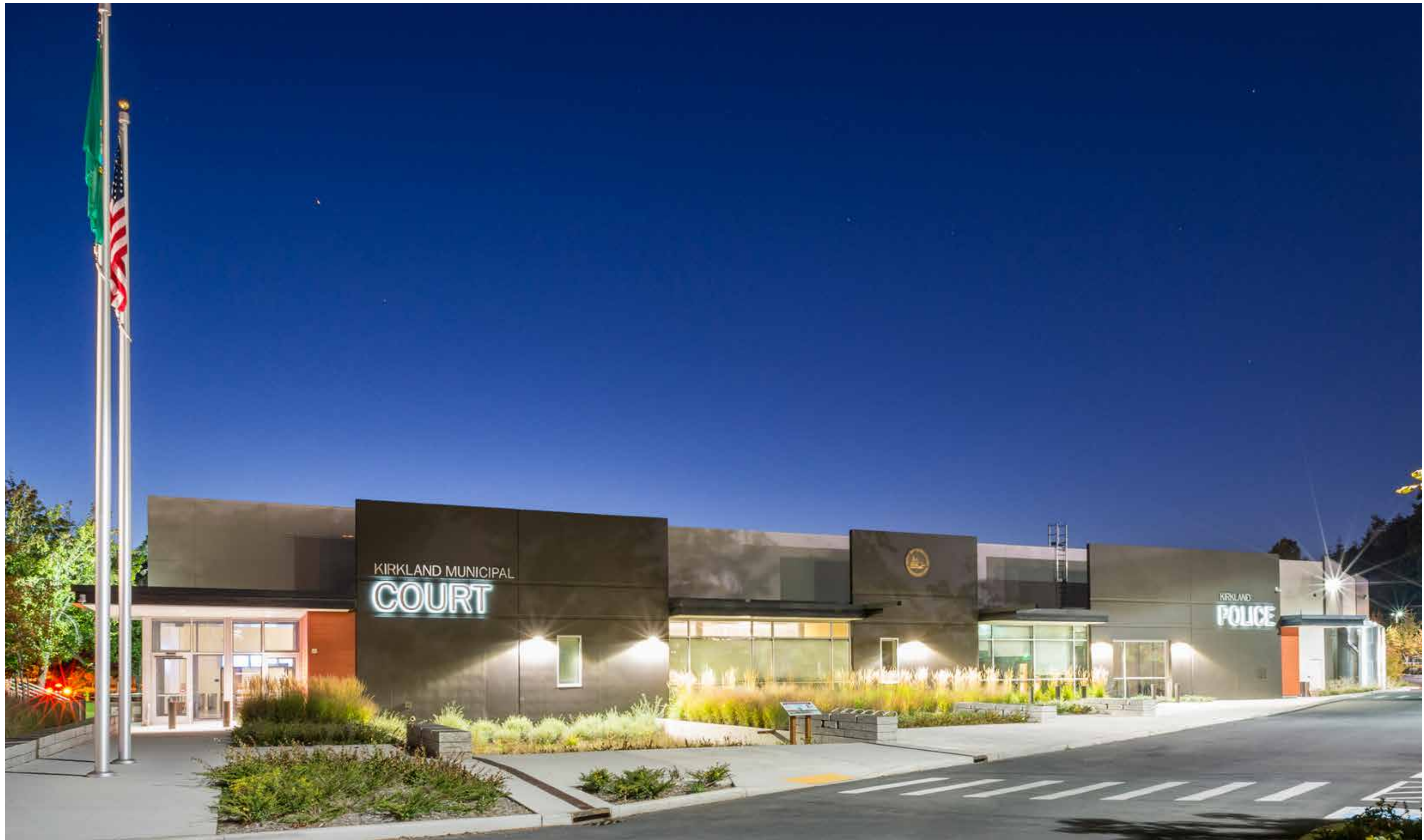
Civic Presence: From a distance the building now clearly possesses a civic presence. Upon arrival, layers are revealed and demonstrate how green stormwater infrastructure (GSI) and material re-use are integral to a sustainable landscape.
