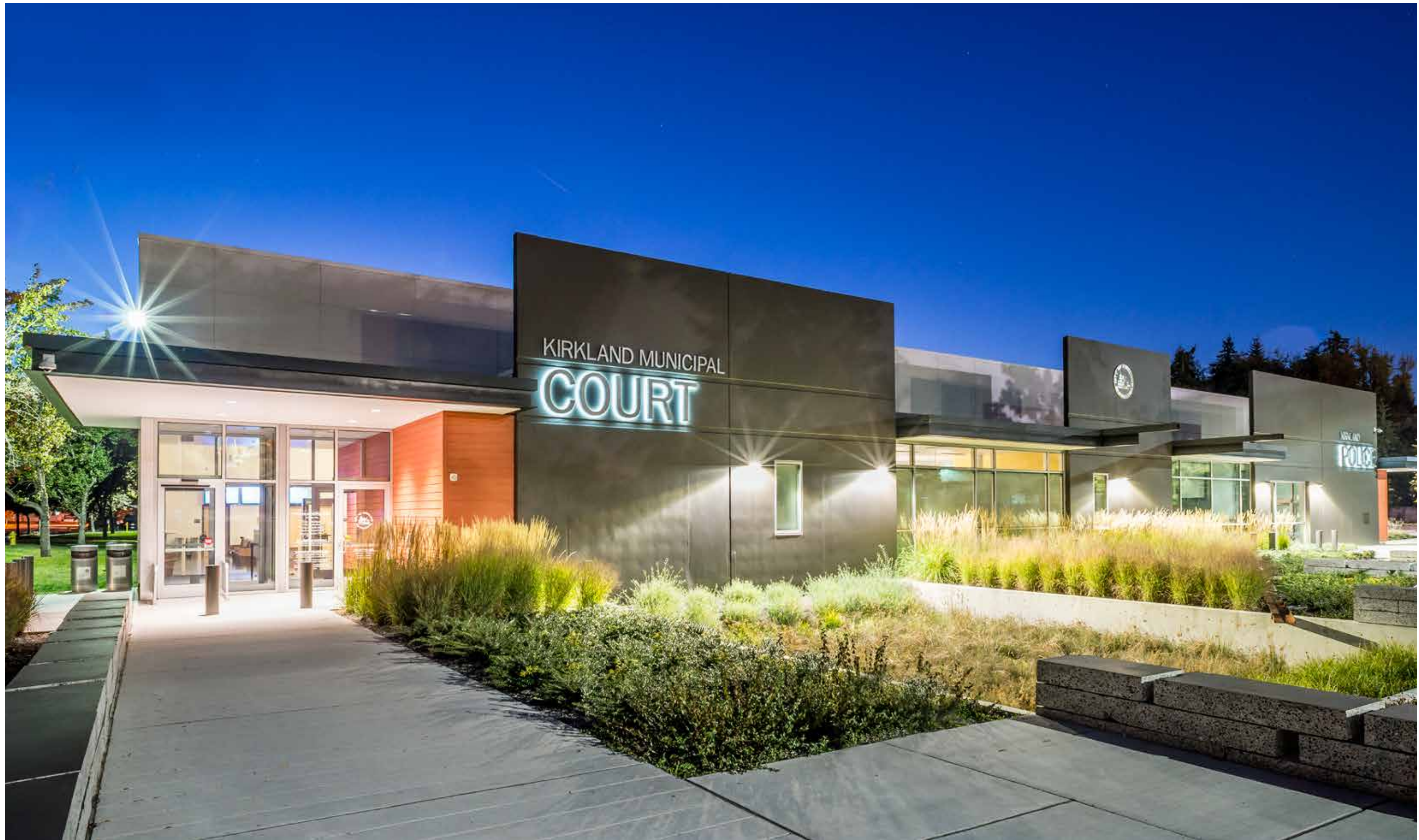
New East Facade: The former back of building is transformed with welcoming civic entries. The loading dock is now a bio-retention planter/rain garden which collects water from the roof while repurposed site walls define the space.
