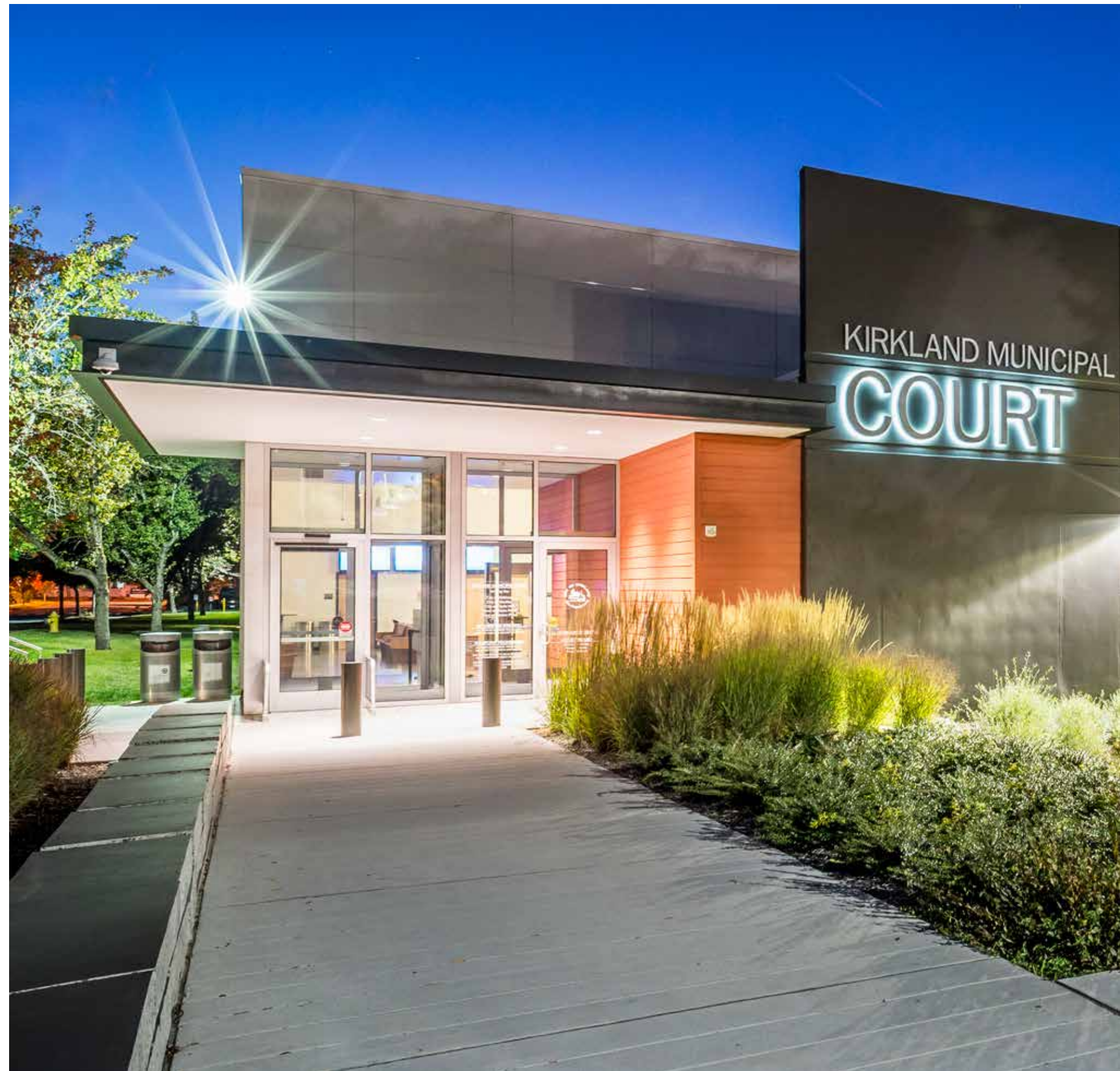
Rescale Entry: Lowering the roof and introducing color, light and planting gives a welcoming, pedestrian scale to the large building.
