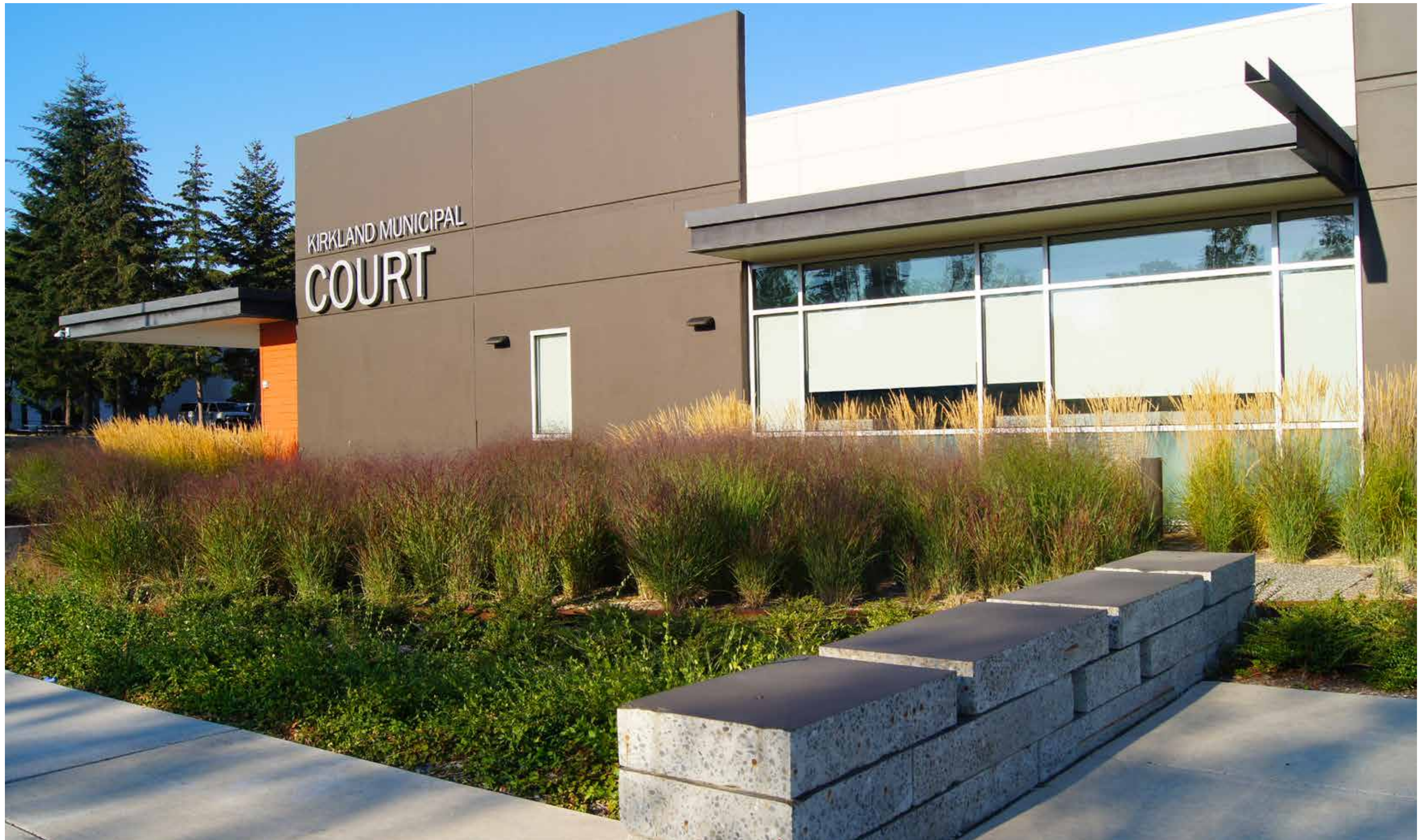
Court Entry: Removed panels and lowered roof change the building's scale. Scuppers celebrate rainwater falling from the roof into splash pads at grade. Runnels direct water toward the bio-retention planter.
